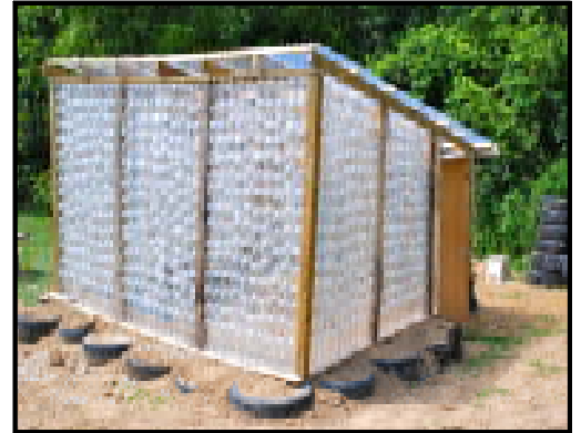
The completed greenhouse at the Mulberry Street gardens.
